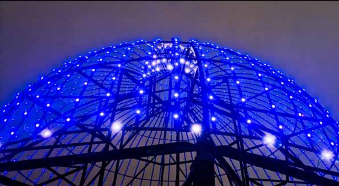
On Aug. 10, 2013, Borisch decided to restore the historical dome on top of McKay Tower, replacing the screw-in incandescent bulbs with roughly 1,200 small LEDs capable of glowing in a variety of colors and patterns as well as producing multiple color-changing effects and animated images.
